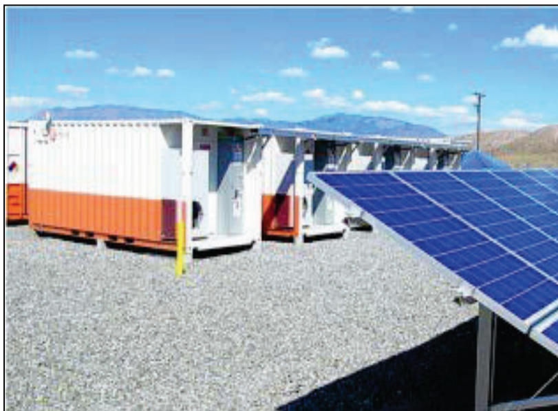
Figure 44. 500-kW/1-MWh Advanced Lead-acid Battery for Time-shifting and 900-kWh Advanced Carbon Valve-regulated Battery for Photovoltaic Smoothing This is a solar energy storage facility that is fully integrated into a utility's power grid. (Source: PNM Resources)
