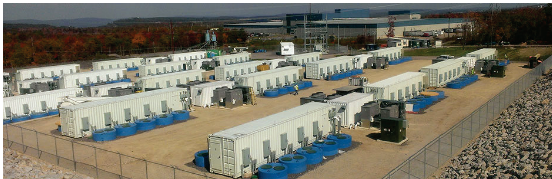
20 MW Flywheel Frequency Regulation Plant (courtesy Beacon Power LLC)
