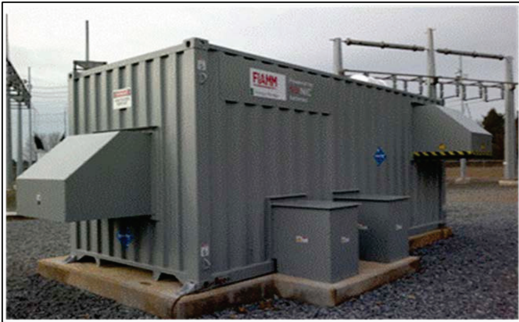
Figure 28. FIAMM 222-kWh System Site at the Duke Energy Rankin Substation
