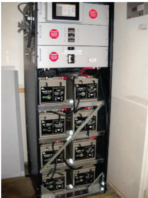
Figure 80. 9.2-kW SP Unit with Cover Removed
