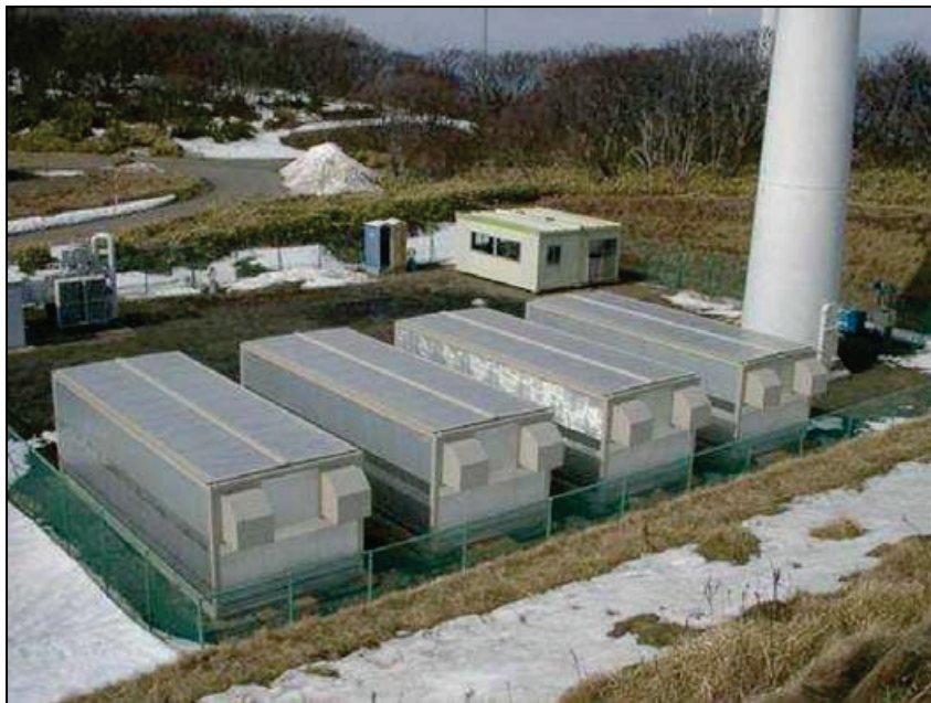
Figure 42. Acid Battery Installation at Tappi Wind Park (Courtesy Hitachi) 4749
