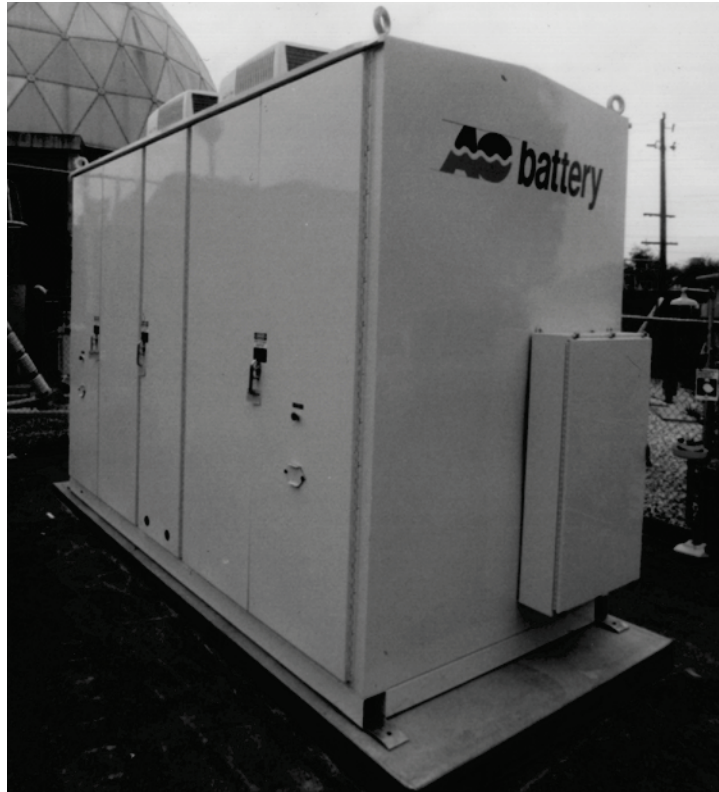
Figure 68. First AC Battery PM250 Modular Battery System Installed at Pacific Gas & Electric's Modular Generation Test Facility, San Ramon, CA, in 1993.
