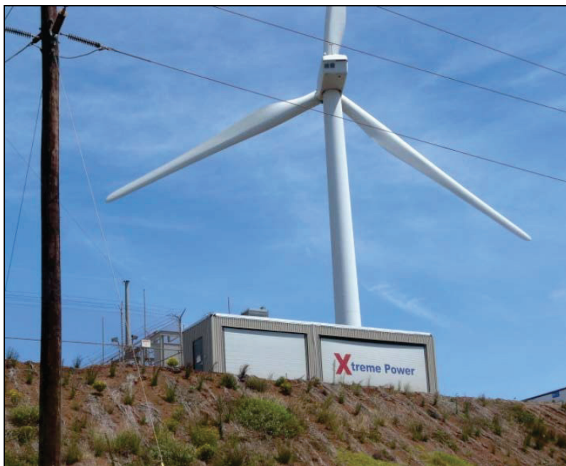
Figure 43. 1.5-MW/1-MWh Advanced Lead-acid Dry Cell Systems by Xtreme Power in a Maui Wind Farm (Source: Xtreme Power)
