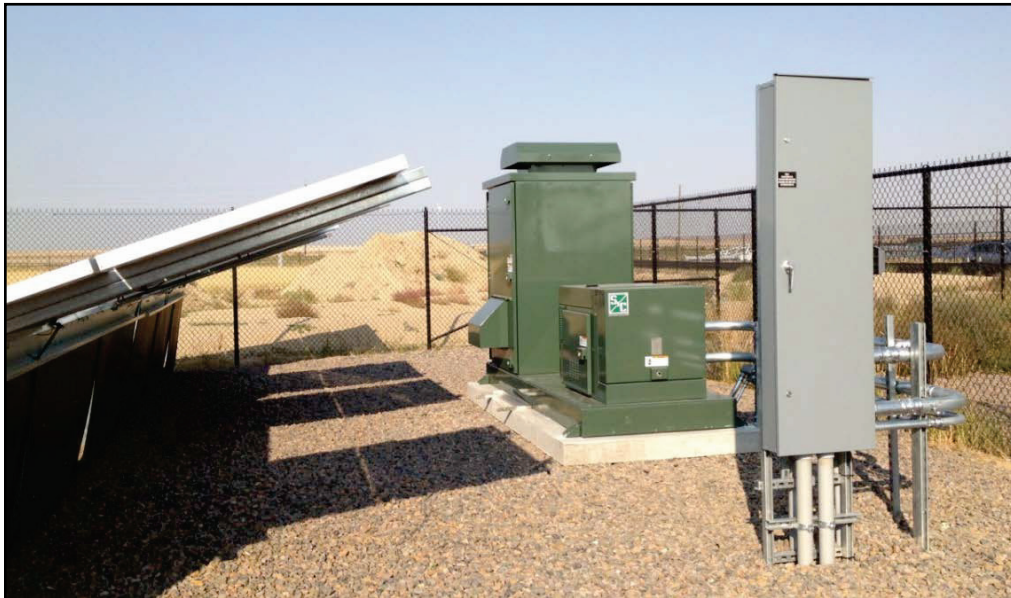
Figure 29. Containerized 25-kW/50-kWh FIAMM Battery Unit (large green housing) on Concrete Pad, Next to S&C PureWave CES (small green housing)
