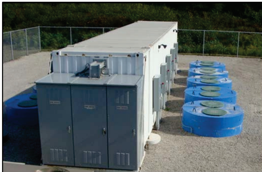
Figure 48. 1-MW Smart Energy Matrix Plant
