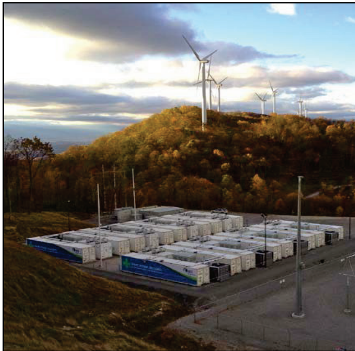
Figure 52. AES Storage LLC's Laurel Mountain Energy Storage (Supplies 32 MW of regulation in PJM using Li-ion batteries supplied by A123 Systems)
