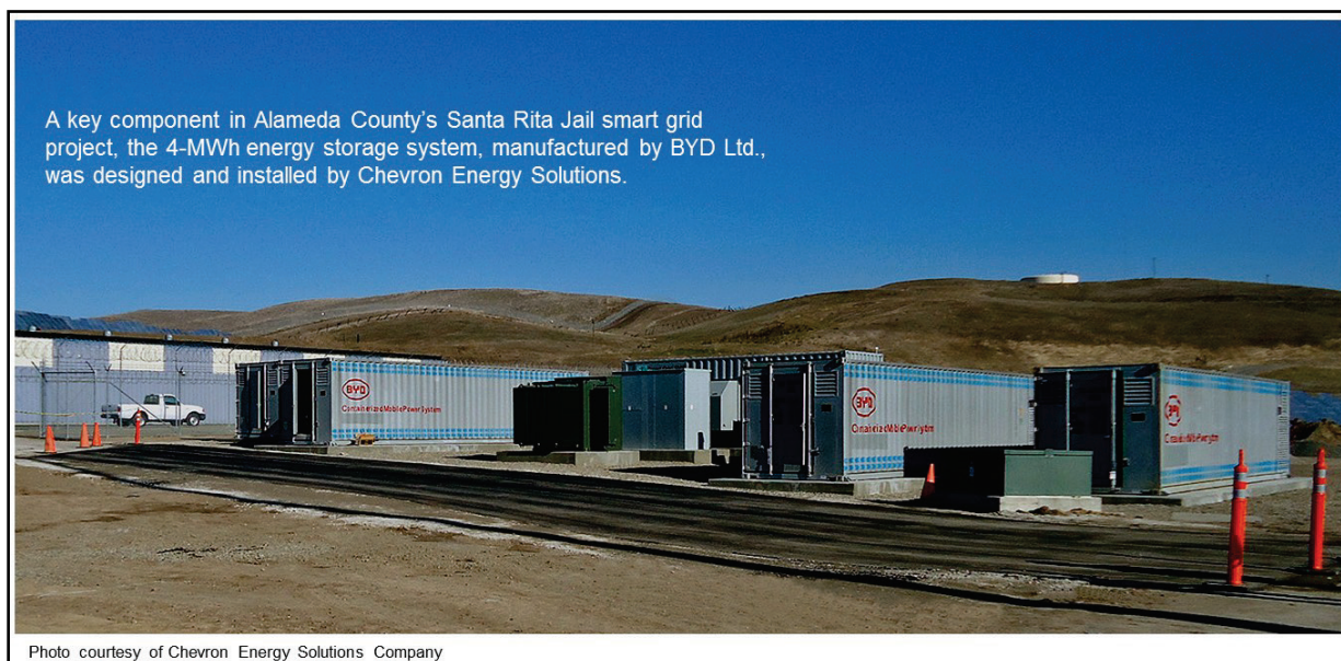
Figure 53. A 2-MW/4-MWh Li-ion Energy Storage System
